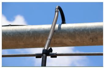
Figure 9. Truss rod hose clamps/slings.
