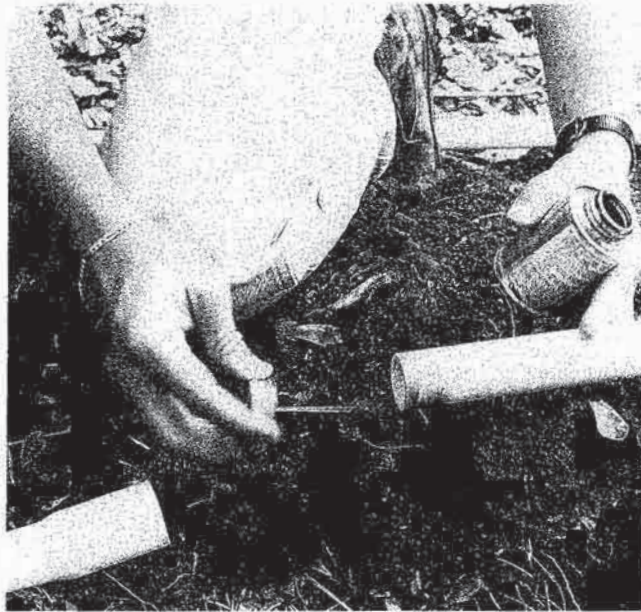
Figure 7.2. Primer and glue application on PVC pipe.
